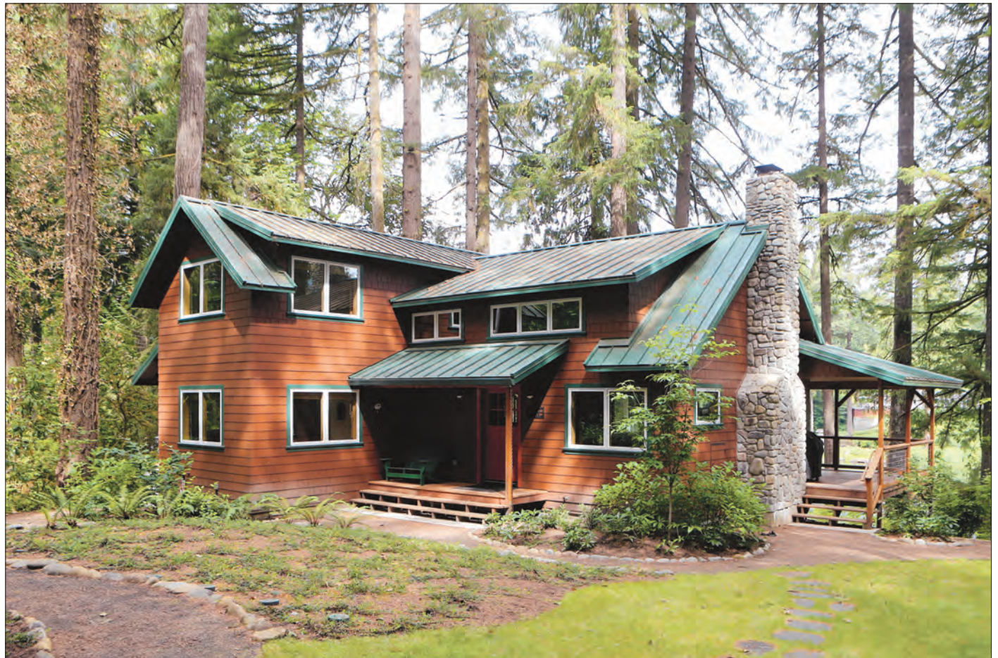
Cement-based shingles in wood pattern and metal roof add to durability and low maintenance; shed dormer’s windows fill living room with light.
