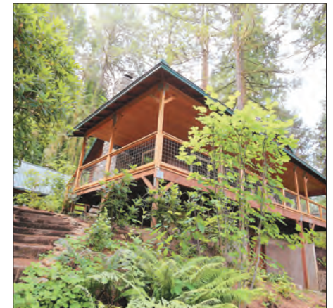
New cabin’s deck has wide hemlock overhangs with beadboard ceiling and hog-wire railing. Steps lead to the dock below.
